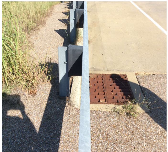
PHOTO 2 Description Abutment 1 erosion around drain.
