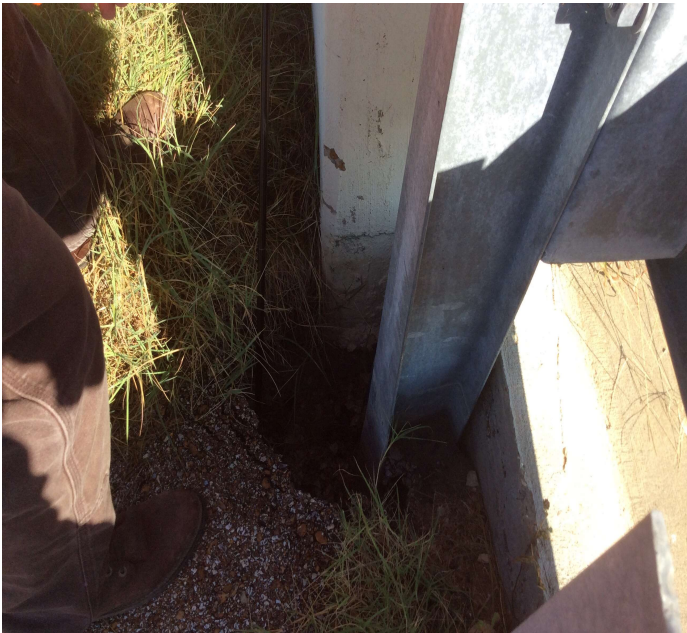
PHOTO 1 Description Abutment 1 left side at bridge rail has 2' deep erosion area.
