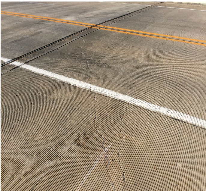
PHOTO 1 Description Approach slab cracks.
