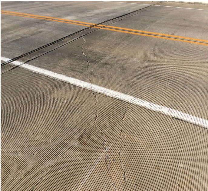
PHOTO 1 Description Approach slab cracks.
